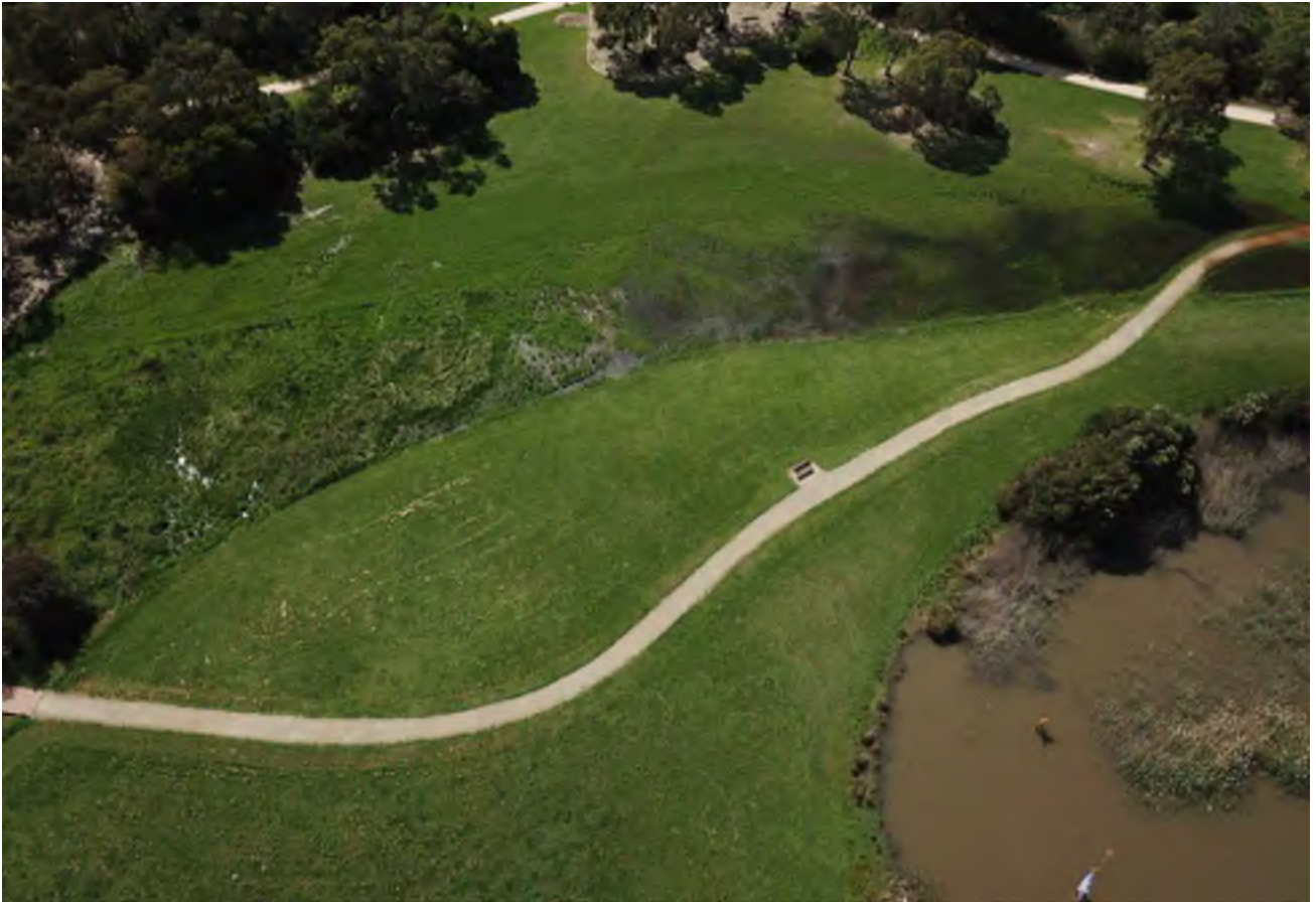
Photo 19. Inundation within drainage-line; Tirhatuan Park (October 2020)
